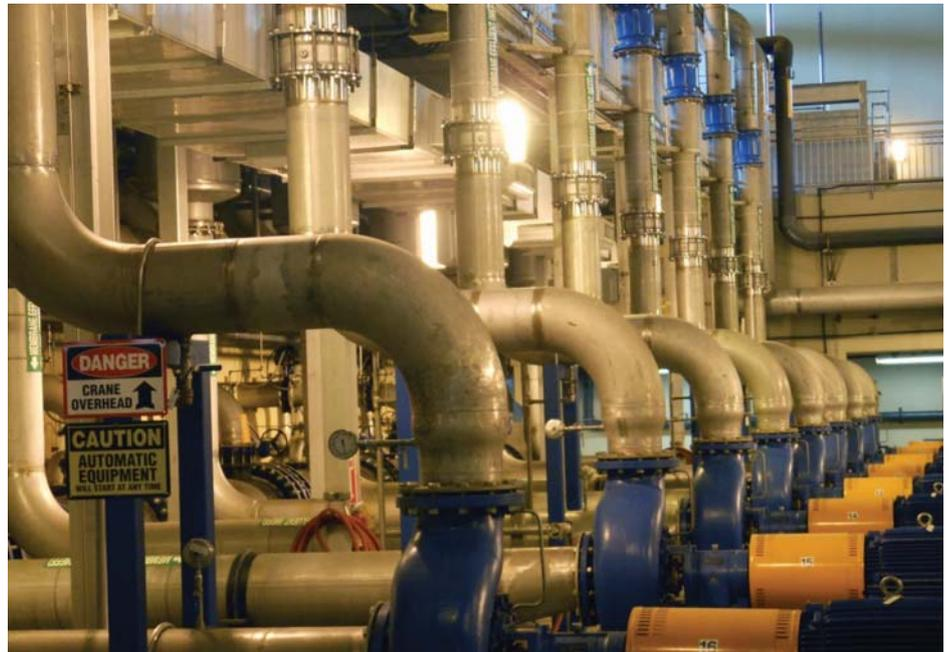
*The current installation updated with DFT axial flow check valves installed in a vertical flow up orientation, eliminating the hydraulic shock/water hammer in the membrane facility.*
